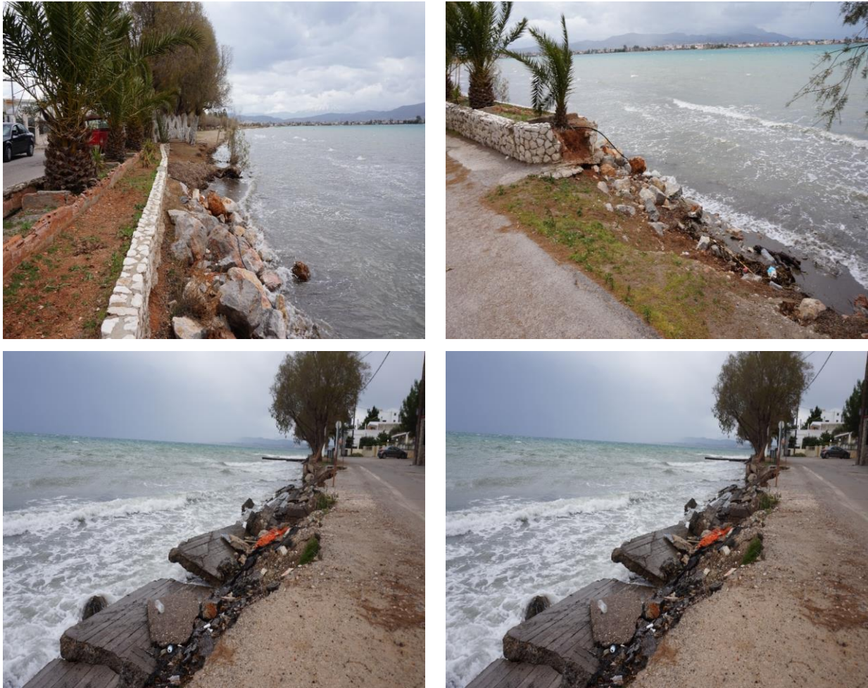
Figure 2. Evidence of damage to the coastal road due to erosion
